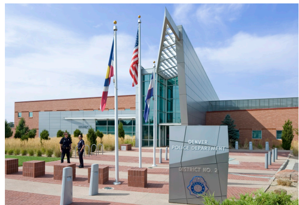
CITY OF DENVER POLICE SUBSTATION NO. 2 Denver, CO
