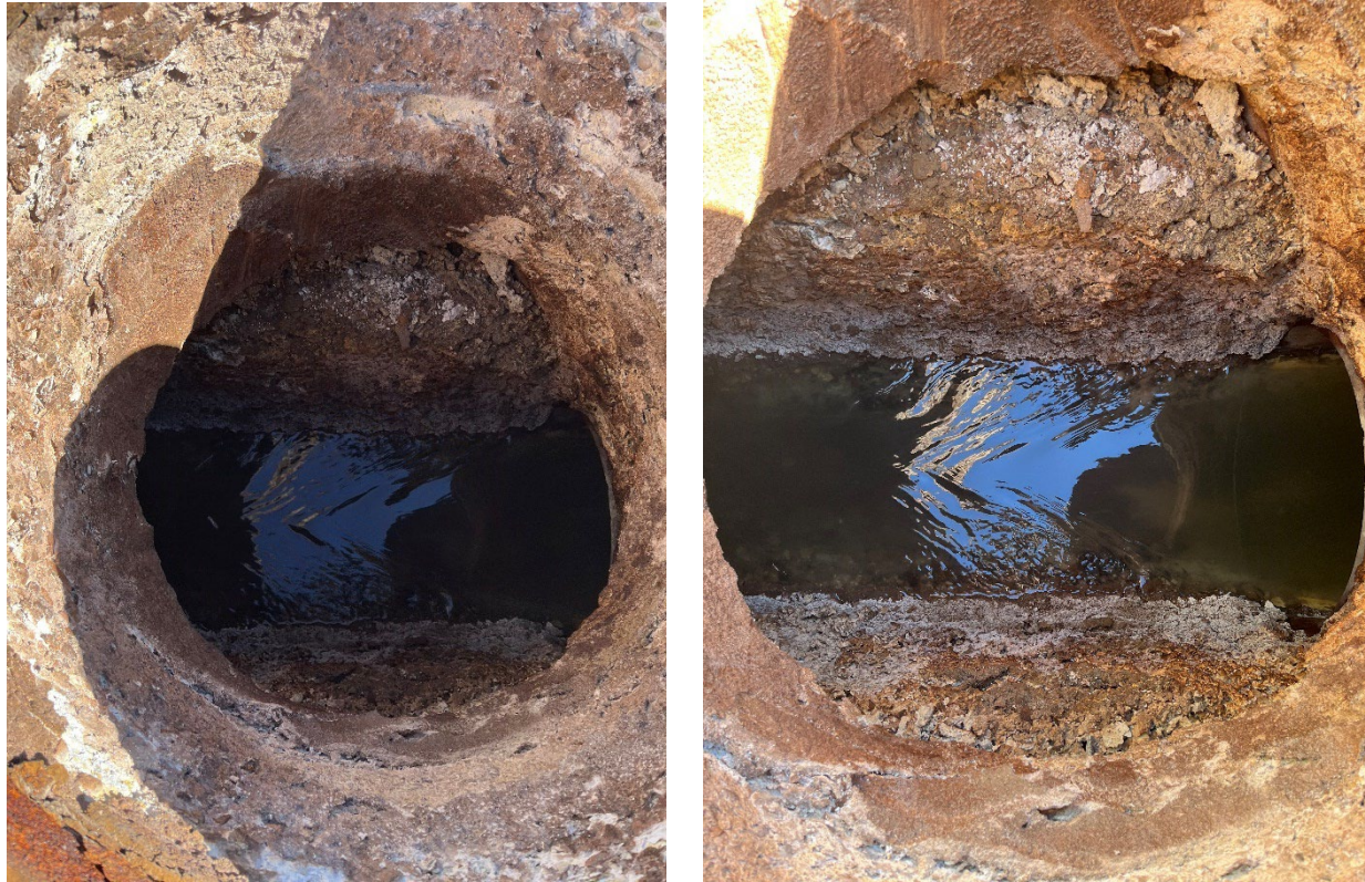
Figure 6-1 Interior of Manhole 7004
