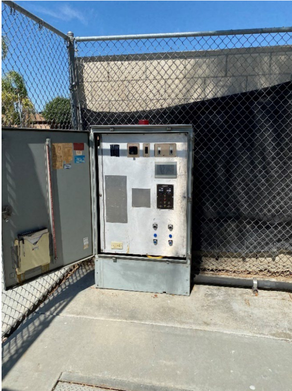
Figure 6-2 Hail & Fifth LS Control Panel and Access Hatch
