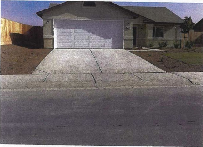
Driveway with rolled curb & gutter
