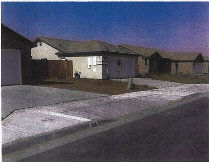
Driveways without rolled curb & gutter
