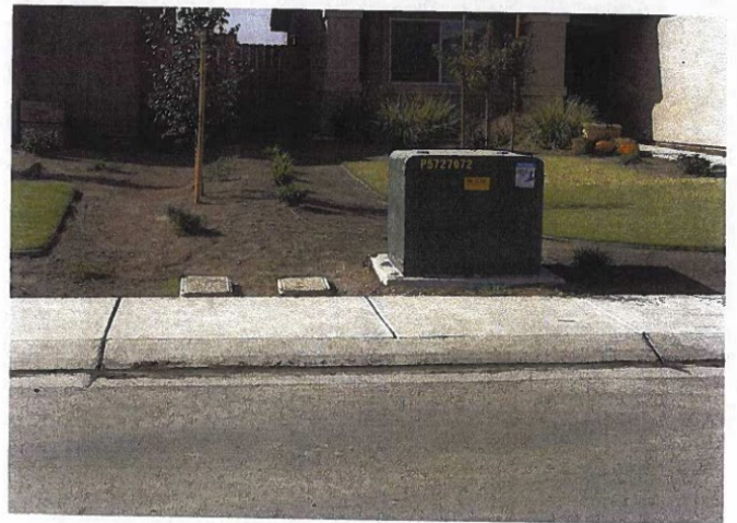
Utility boxes with rolled curb & gutter
