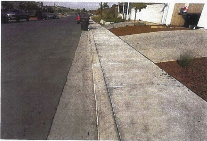
Rolled curb & gutter
