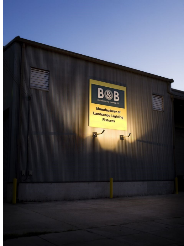
Figure 42. These up-lighting fixtures serve to brighten, bring attention to, and emphasize the architectural form of this façade. Note how the light pattern enhances and reveals the pattern on the steel and concrete due to effective fixture placement and use.
