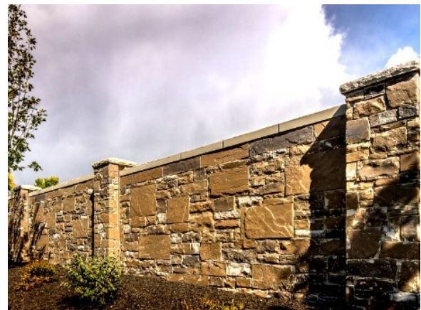
Figure 26. Note the use of pilasters and caps to add variation to this wall. Also note the use of baffling in the form of mixed stone and landscape to reduce noise reflected while providing an effective security barrier.
