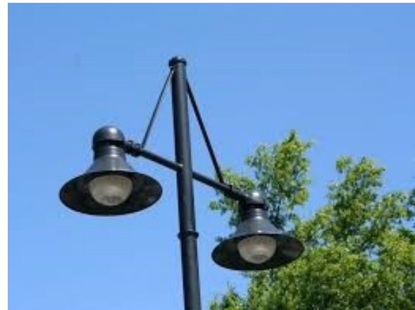
Figure 40. Decorative, shielded lighting fixtures help increase security and safety for pedestrians onsite and prevent light spread to other properties.
