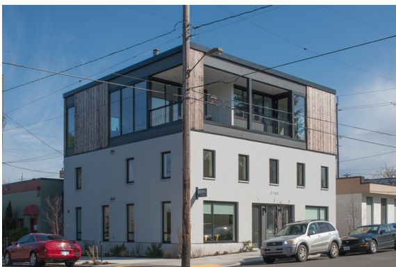
Figure 13. Atypical design elements help increase interest and engagement, while street-facing pedestrian entries increase visibility, comprehension, and neighborhood compatibility.
