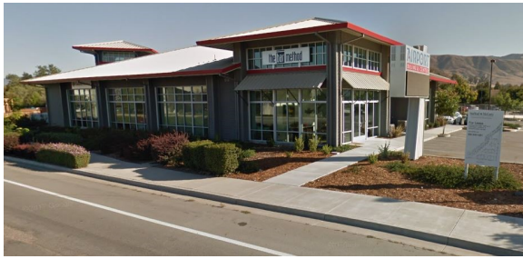
Figure 3 - Buildings sited toward the street with connected paths that access sidewalks increase legibility, safety, and value of the property.
