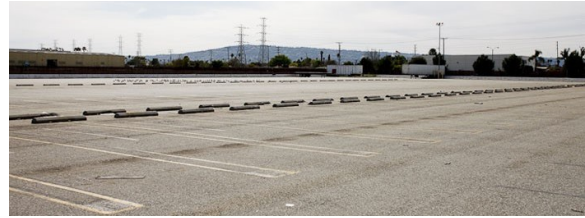
Figure 37. Do not design sites with empty, bare parking lots. These act as heat islands, increasing costs and injury risk for users. Redevelopment projects: add landscape, berms, or shade to provide variation and cover.
