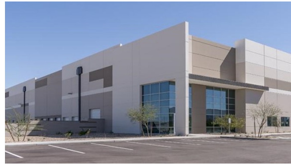
Figure 16. The Tolleson Logistics Center, a new Class A industrial site in Arizona, demonstrates the principles of breaking the sight line through vertical and horizontal material differentiation, recesses into the wall indicating the main pedestrian entrance, and landscaping that separates the parking area from the main building. Other buildings can achieve the same effect through use of varied metal articulation or alternate blocks and patterns of paint. Note also that functional elements such as the drain downspouts on the left wall break up the shape and form of the building, and the strong color contrast between dark blue downspouts and the desert-tan shades of the building act to provide visual relief. Further, the loading area seen to the left, well screened by a wall and differentiated from the main entrance while still physically near the industrial office, draws visual interest with windows.
