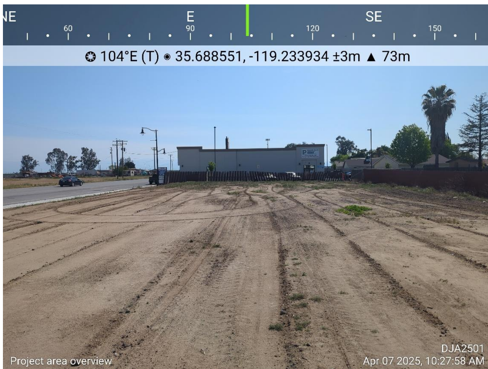
Photo 2: Overview of Project Site (View E)
