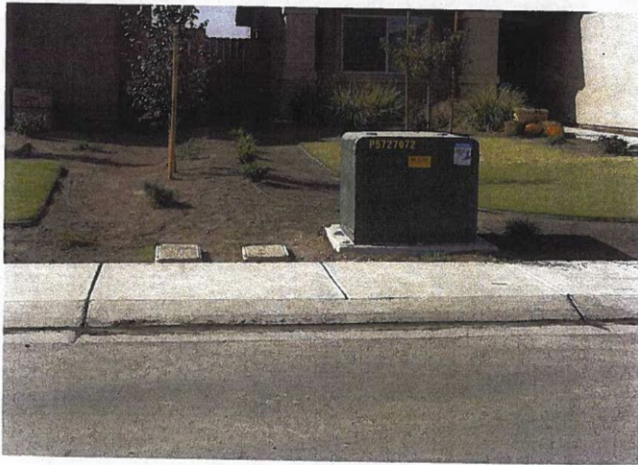
Utility boxes with rolled curb & gutter
