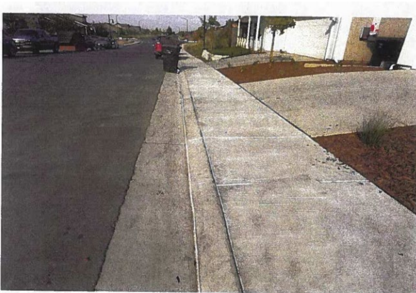
Rolled curb & gutter
